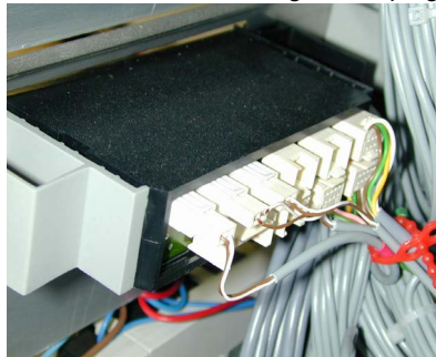
Fig. 4: Connections for pre-assembled cables
