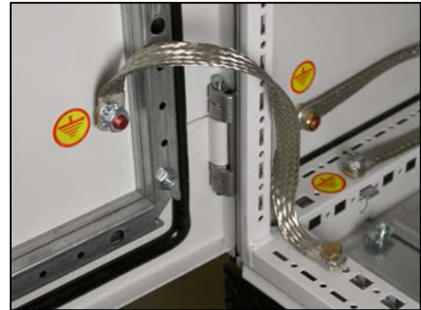
EMC-appropriate earthing with a highly flexible earth band
